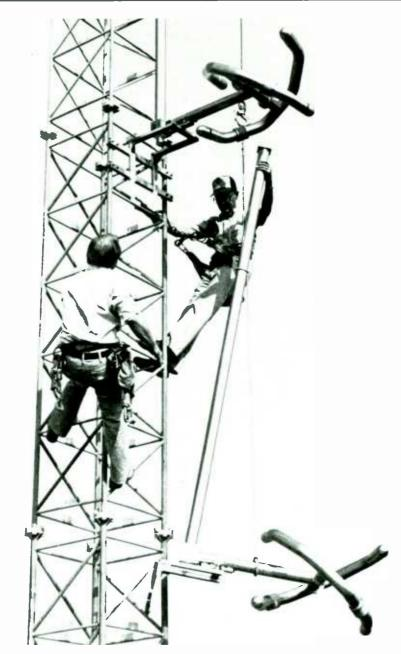
dipoles are constructed of 3-1/8" o.d. brass which provides an excellent element bandwidth as well as protection against corona discharge failure.
